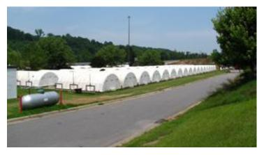
Figure 1. Rotating Biological Contactors
